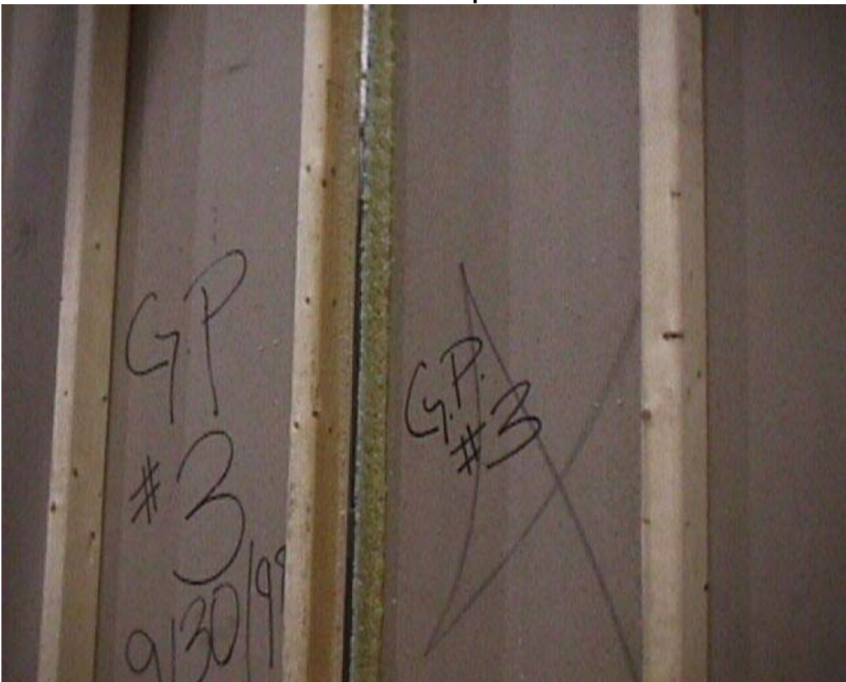
Test No. 3 at Failed Area
