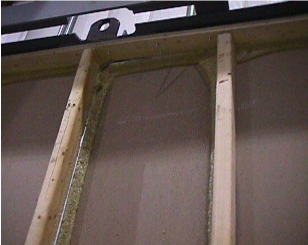
Test No. 1 at Failed Area
