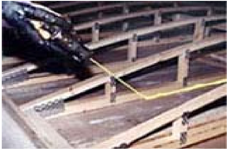
Figure 3 - Typical Spray Application
